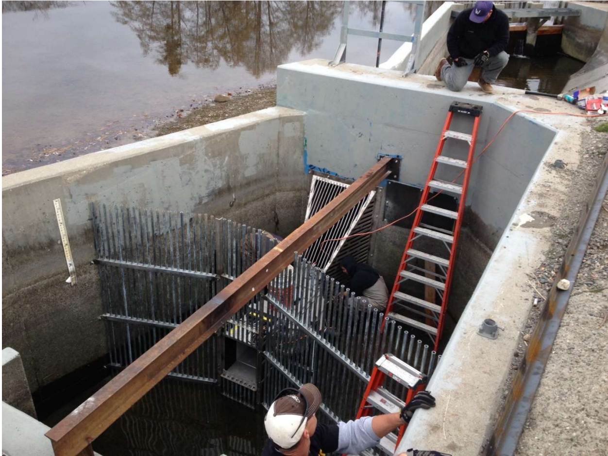
Figure 25. VAKI Riverwatcher installed in the fish ladder adjoining Durham Mutual Diversion Dam.
