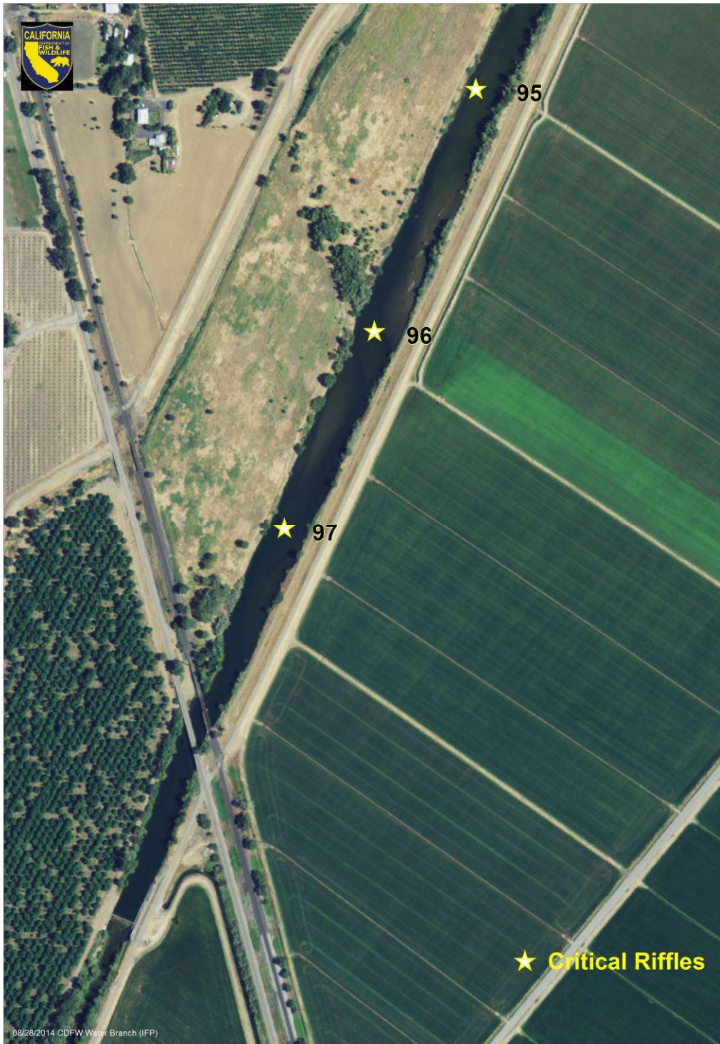
Figure 18. Critical Riffles 95, 96, and 97 upstream of Midway Road with the flashboards in-place at Gorrill Diversion.
