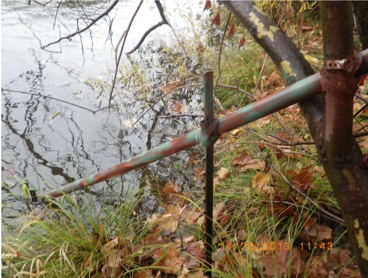
Figure 24. Pressure transducer mounted in PVC casing downstream of Lahar site.
